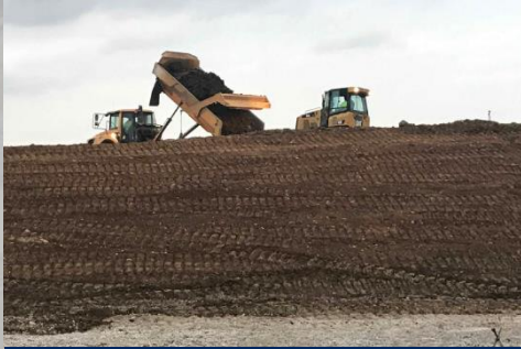
Construction of P1 Surcharge
