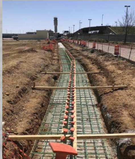
Excavation & Construction of Blast Wall
